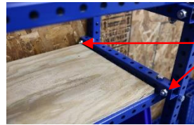
Fig. 1 OSB Sheathing for shelves may be placed in position without mounting. Bolts connecting frame will naturally hold in place
